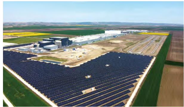
PV power generating system at our Serbia Factory
